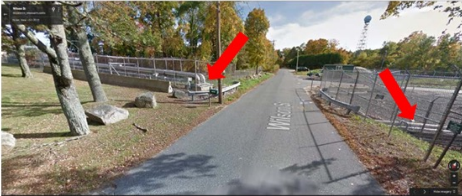
Figure 1. Image of the pipeline road crossing under Wilson St. at the NSTAR facility. Note that any LNG spill from the pipeline will collect in the depression on the right side (west) of the road. Arrows indicate the pipeline impact point identified by Smith & Burgess and the depression.
